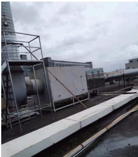
Exhaust Gas Treatment at Dongguan Fuyang Plant: Two-stage Activated Carbon Box
