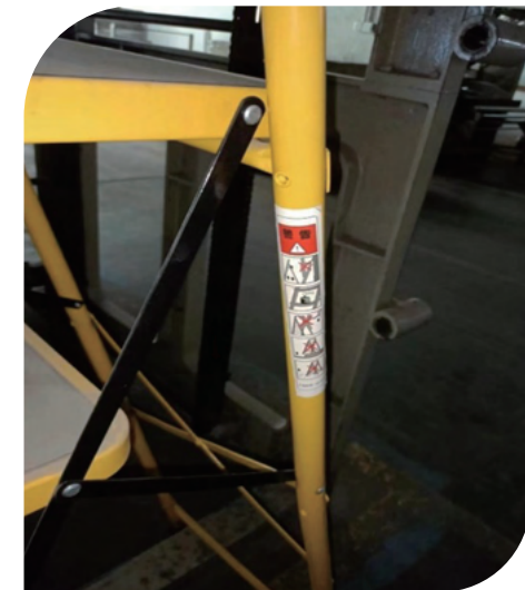
Posting of safety warning notices at conspicuous places on escalators
